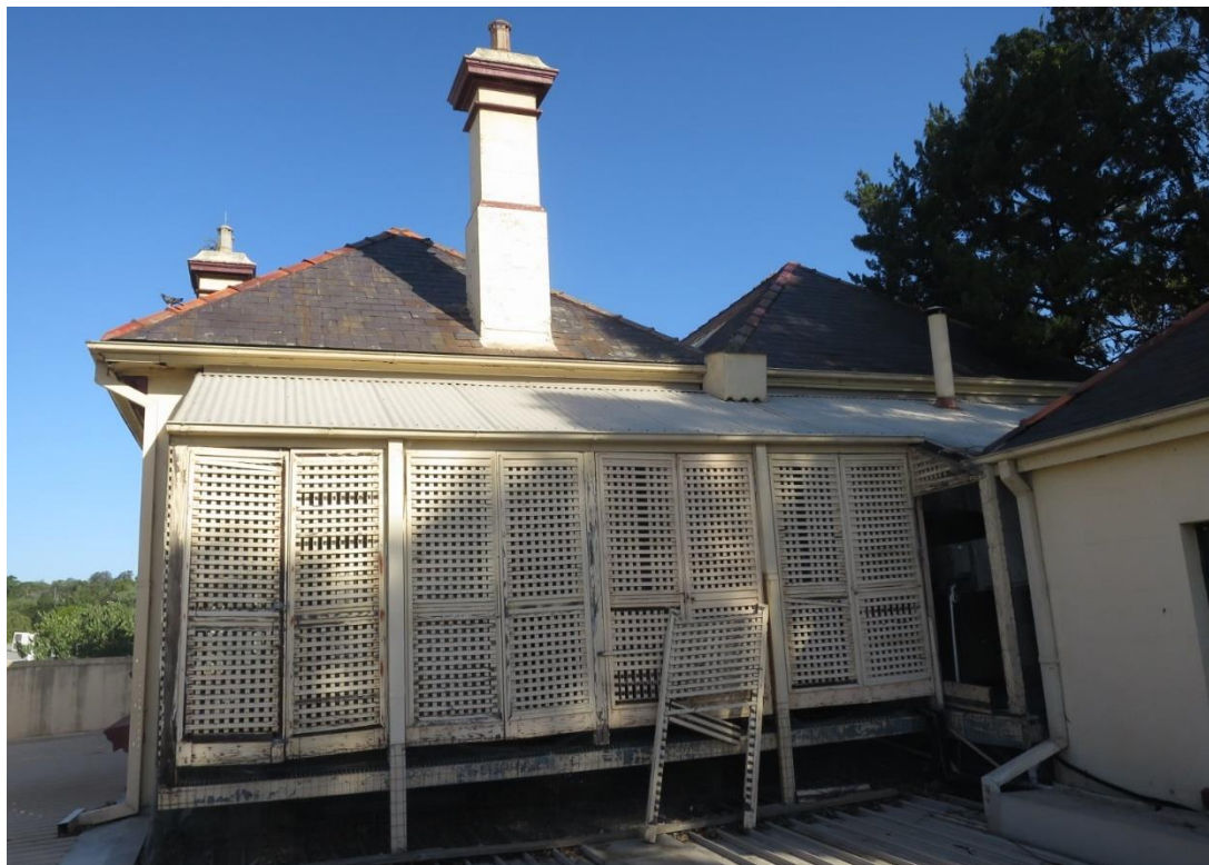
Figure 22 – the rear veranda is from the 1985–95 period. It screens the air-conditioning equipment. NBRSArchitecture February 2017.
