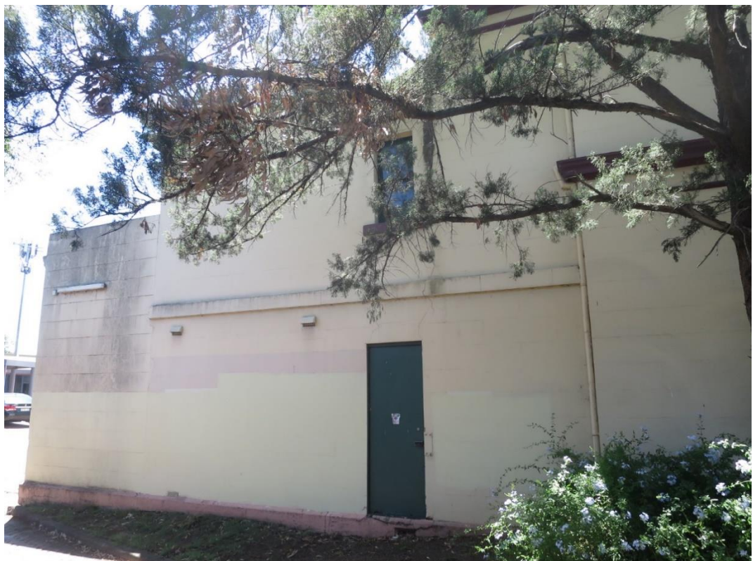
Figure 18 – the south-west elevation of the remains of the service wing. The two-storey section is original, but altered. The single-storey section on the left is 1990s fabric on the site of the much longer single-storey service wing that contained the laundry and coal stores. The tree is a Virginian juniper. NBRSArchitecture February 2017.
