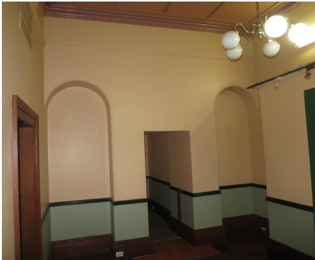
Figure 30 – the original dining room G.05 on the ground floor. The niches, skirting and cornice are original, but the central fireplace has been turned into a doorway to the former strong room. The chimney rises over the left niche.
