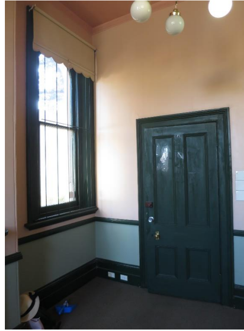
Figure 26 – original door and side elevation window in G.03 to be replicated in the conservation works.
