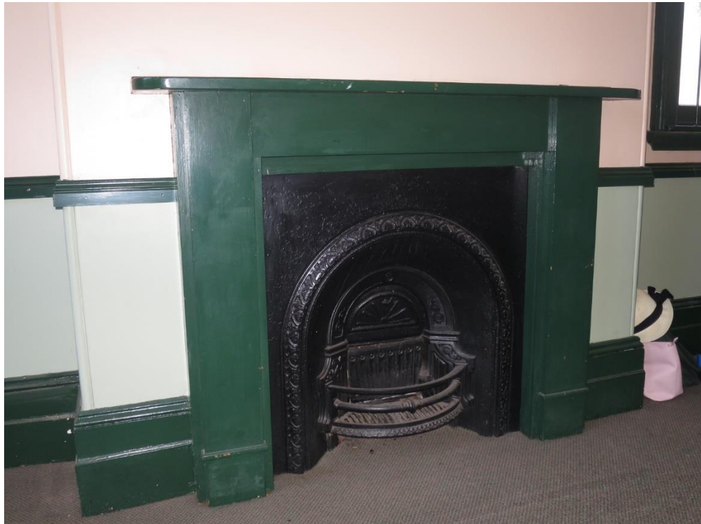
Figure 27 – likely original cast iron coal grate in G.03. the timber mantelpiece is recent and should be replaced with a Victorian design in marble. NBRSArchitecture February 2017.
