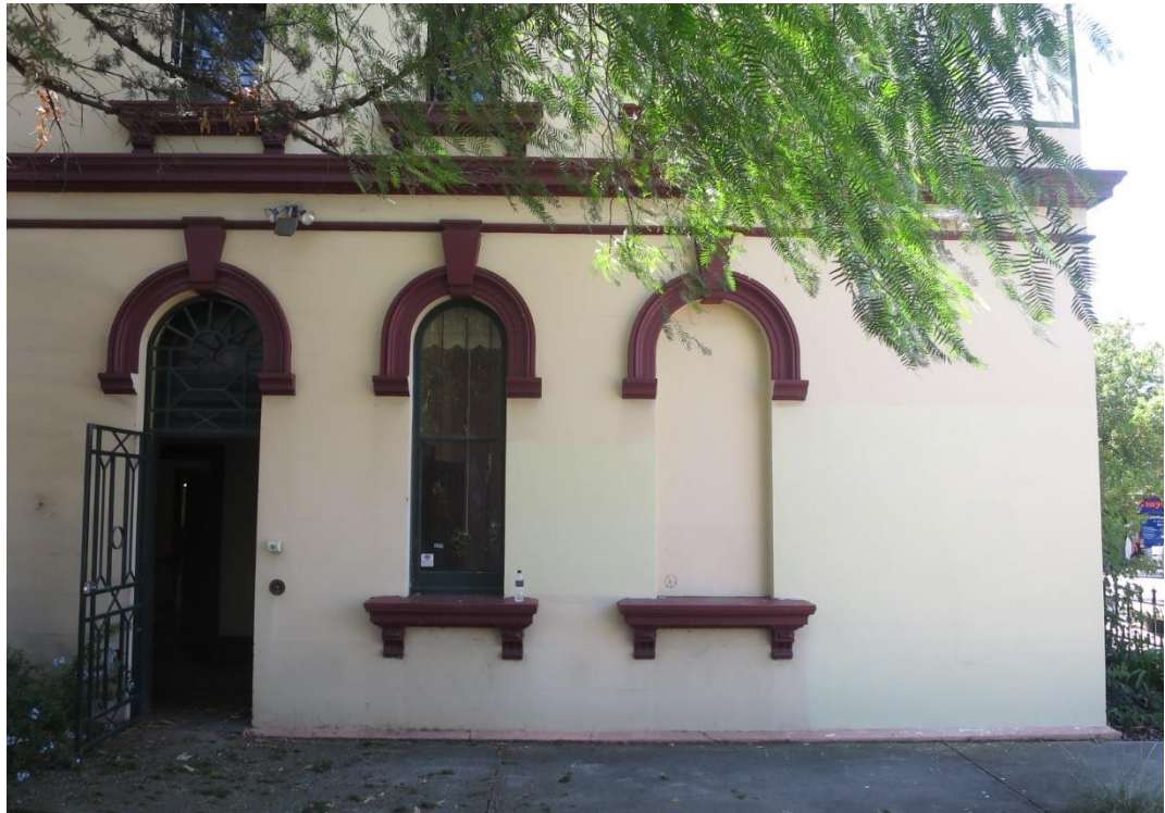
Figure 17 – the entry to the residence and window of the bank manager's study on the south-west elevation. The timber door is original. NBRSArchitecture February 2017.
